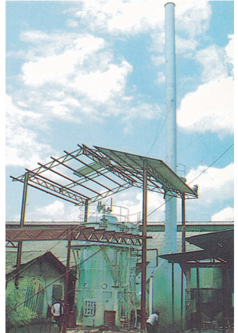
Site installation in progress
